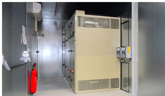
E-House equipped with MBS
